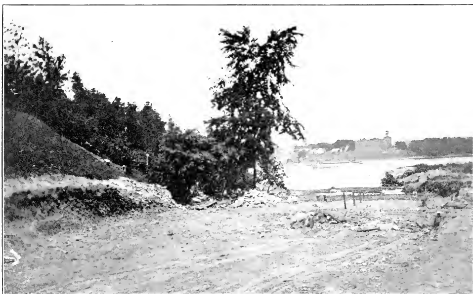
Entrance to Lady Grey Road (under construction).
