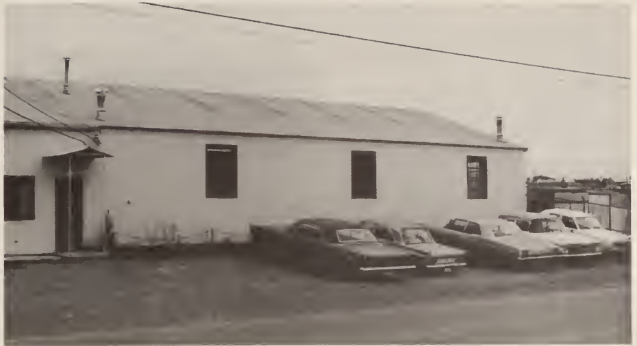
The Precut Building Plant in Calgary
