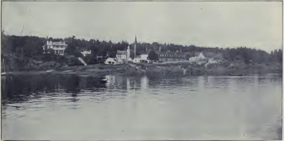
QUARANTINE STATION AND BUILDINGS, GROSSE-ISLE
